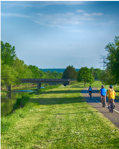
Water management and mobility in the same corridor.
